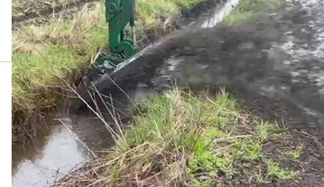
▲ High pressure ditch maintenance
